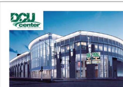
Digital FCU [Named this arena] Marlborough, MA Assets: $3.5 Billion
